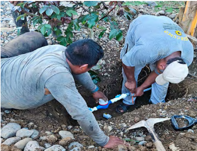
At the request of the communities, we began a pilot project to install home water meters in Huacaria and Shintuya to promote equitable access to clean water.
