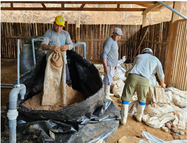
Critical repairs were made to the water infrastructure by the water committees, restoring water to 500 people in Yomybato.
